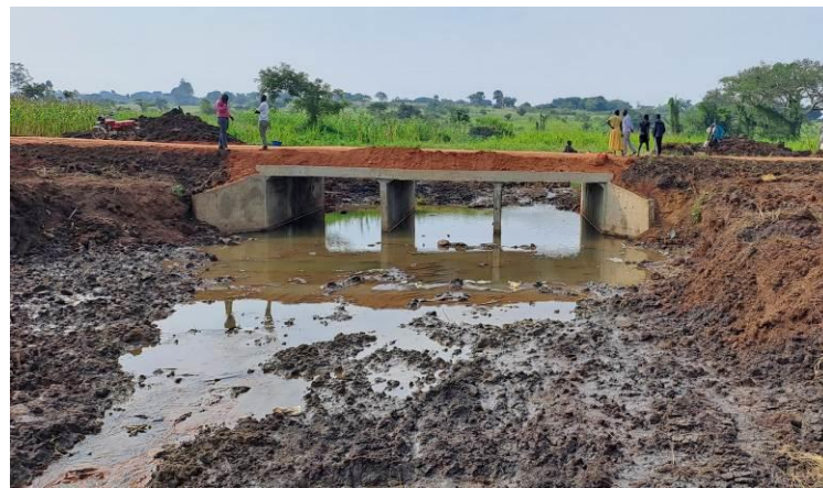
Akago River before and after construction of the box culvert
