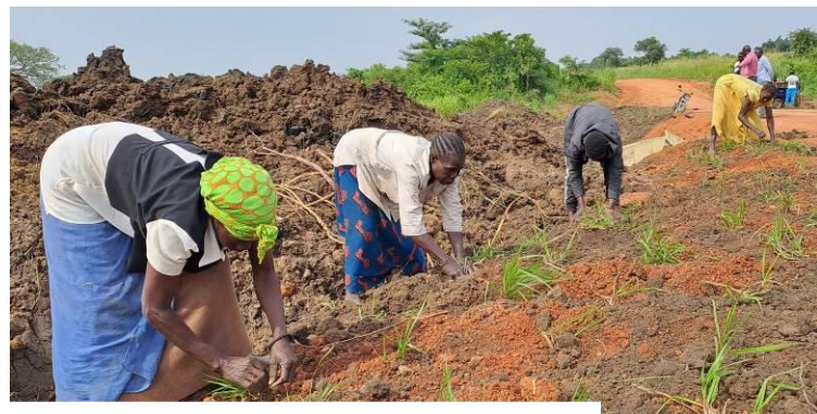
Grass planting at Ogonyi (Left) and Akago (Right) for soil stabilization around the culvert
