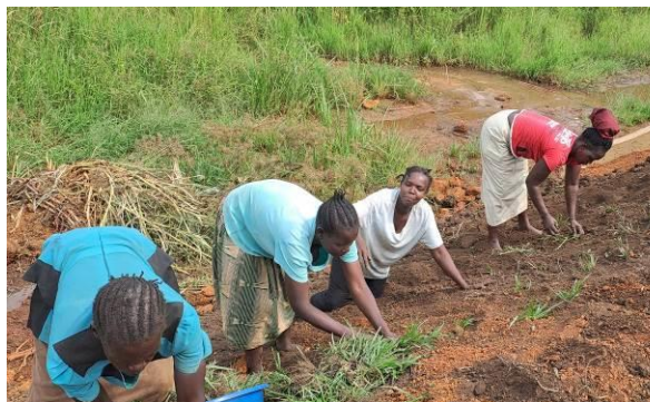
Grass planting at Ogonyi (Left) and Akago (Right) for soil stabilization around the culvert
